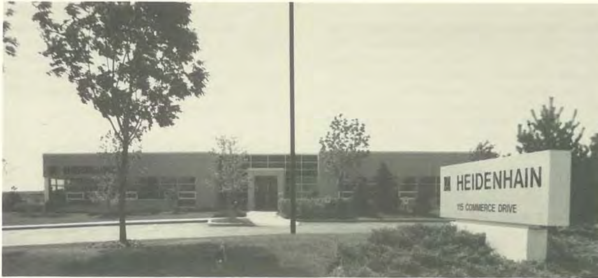
The M-P Zoning District is tailored to facilities operating light assembly, warehousing, industrial/office and research and development functions. Large parcel Industrial/Office uses such as the Heidenhain development are typical of one and two story development found throughout the Woodfield Business Center II.
