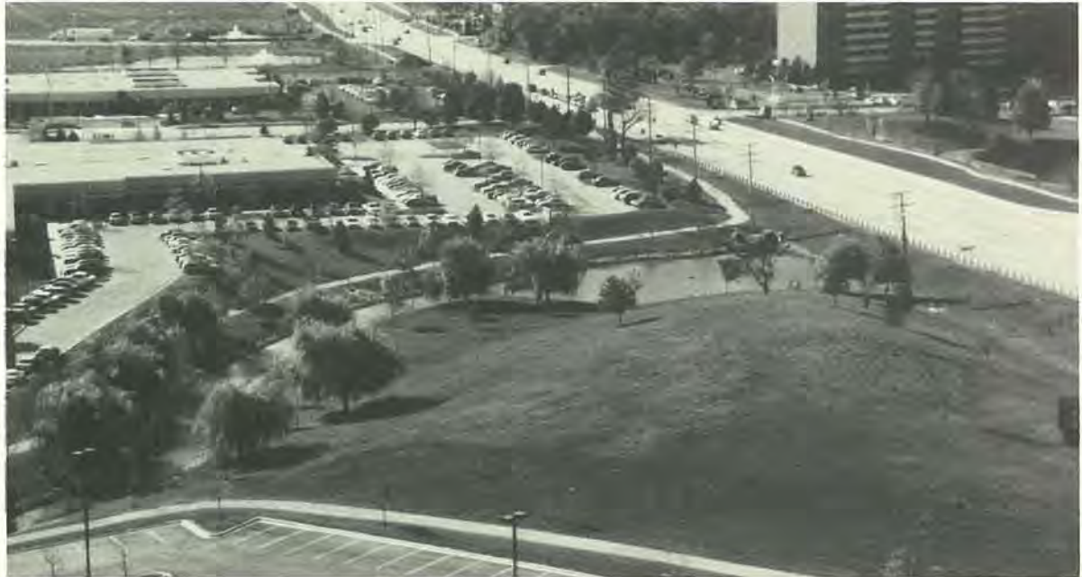
Drainage improvements constructed in conjunction with development of the Woodfield Business Center II were designed to serve as both physical and visual amenities for the subdivision. The Design Guidelines for the Woodfield Regional Center encourage the use of contoured slopes, site furnishings, cobblestone banks, landscaping and other site fixtures to provide for the use of drainage improvements as water features.
