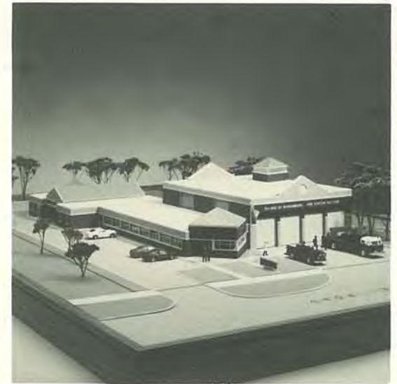
Some public uses, such as Fire Station No. Four, are permitted under the M-P Planned Manufacturing District. The new fire station will be located northeast of the intersection of Amanda Lane and Roselle Road.
