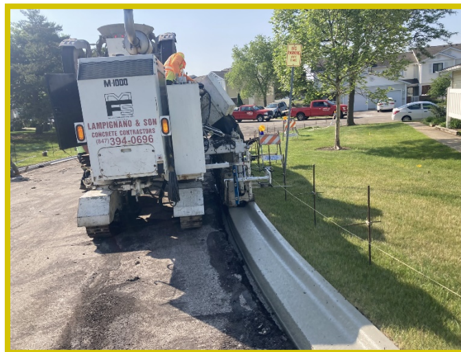
Curb work completed as part of the FY 23/24 Curb Replacement Program
