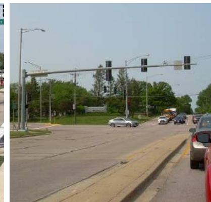
Traffic signals at Meacham Road and Algonquin Road, standard aluminum
