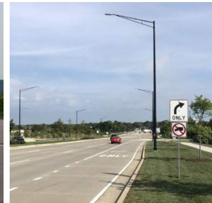
Unsafe pedestrian crossing mid-block between Zurich and Hotel
