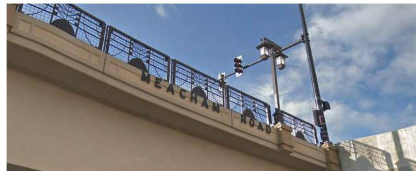
I-90 bridge with prairie style aesthetic upgrades
