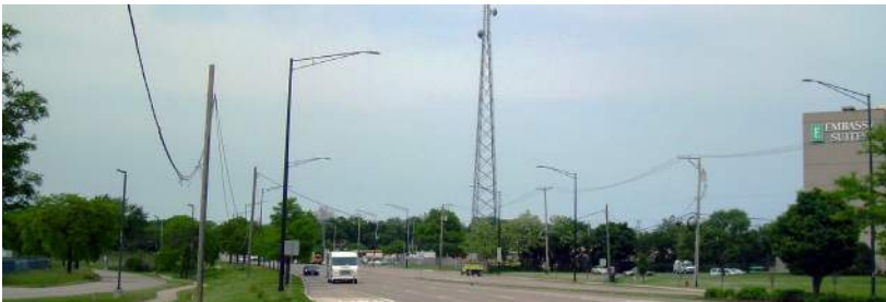
Existing overhead utilities on east side of Meacham Road
