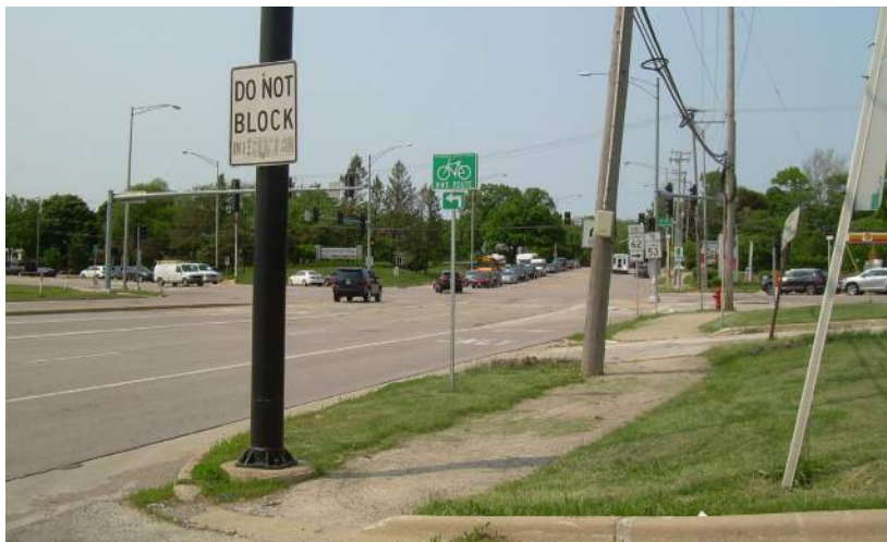
Limited right-of-way to accommodate multiple components
