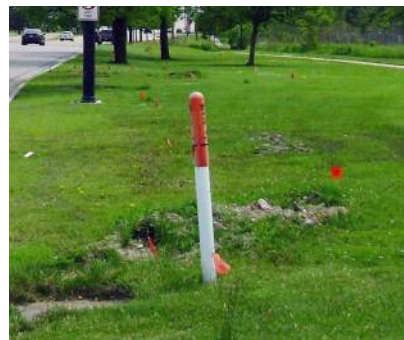
Located underground utilities that must be considered
