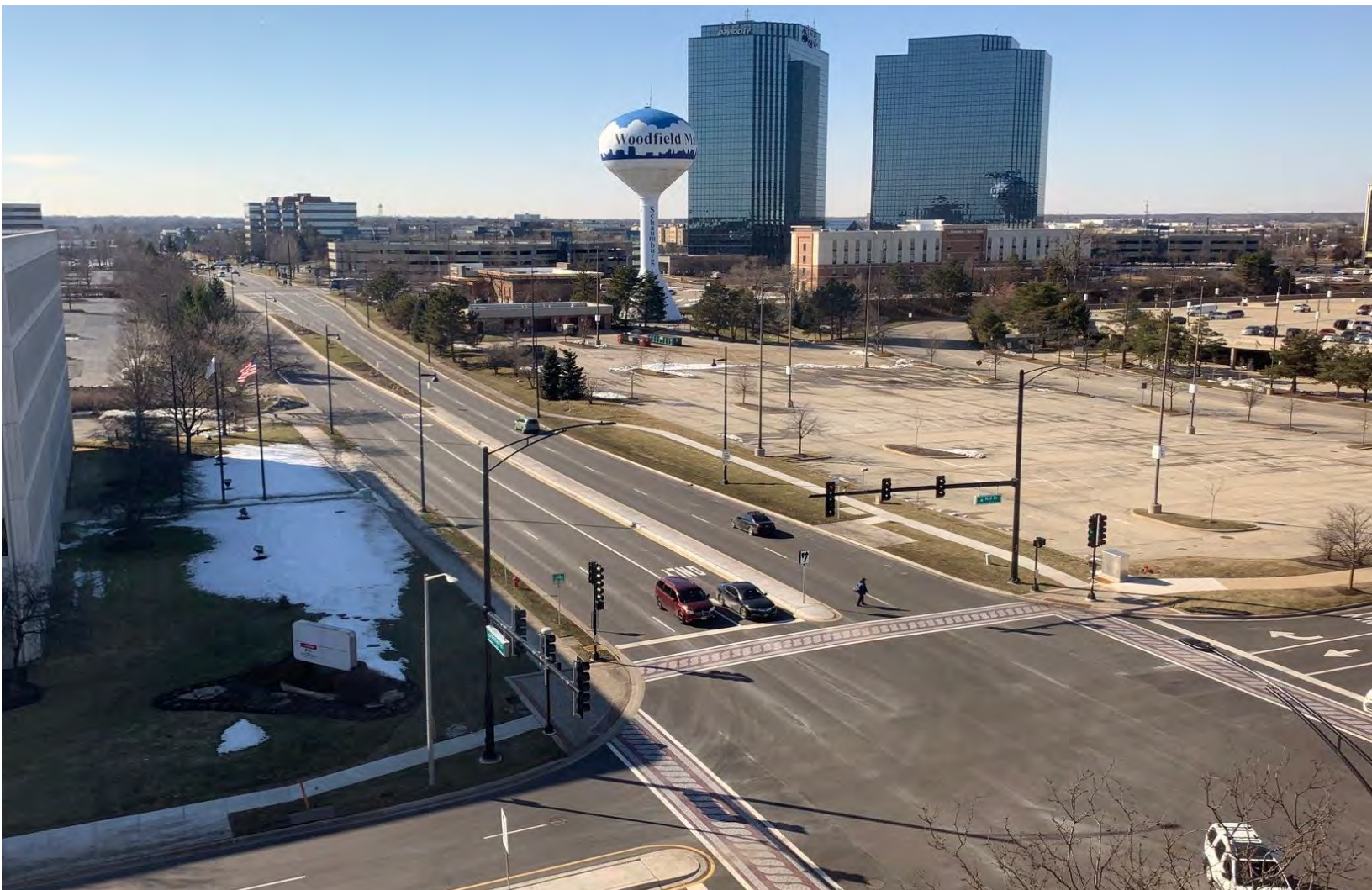
Woodfield Road Reconstruction Project, Completed in FY 2020/21
