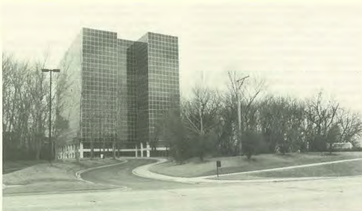
Existing trees at Schaumburg Corporate Center were preserved as a natural feature for the site which also provides a dense wooded buffer for the residences to the south.
