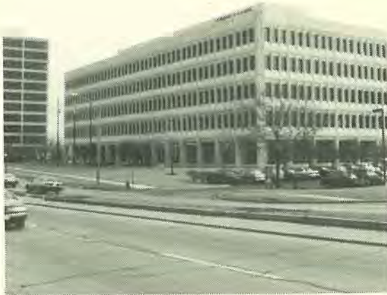
These existing sidewalks on the south side of Woodfield Road will need to be replaced or widened to serve as bikepaths according to the Village's Bikeways Plan.
