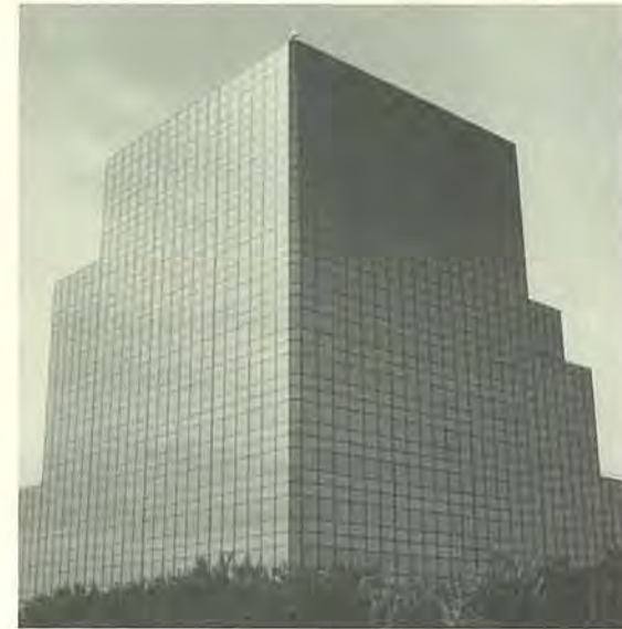
The Centennial Center is representative of the office building boom of the 1980's, the decade when the three office towers within the Unocal Sector were built.
