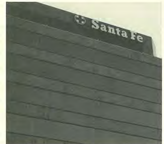
Santa Fe moved into the Century Centre II tower in 1991 bringing its 725 person work force to Schaumburg.
