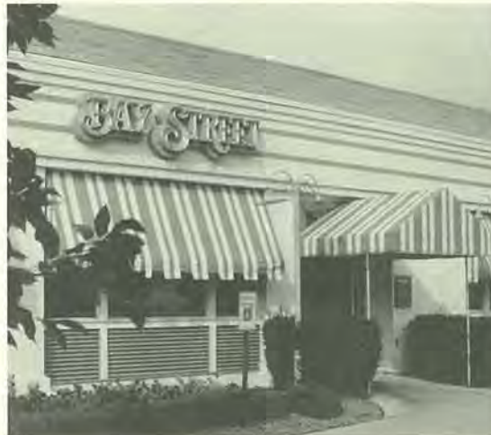
Bay Street Restaurant, located adjacent to I-290, takes advantage of this location as 142,000 cars pass by each day.
