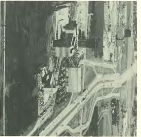
Taken in 1985, this aerial photograph shows Woodfield Corporate Center IV under construction. Note the Fredrickson Farm property to the south and the undeveloped One Schaumburg Place site to the north.
