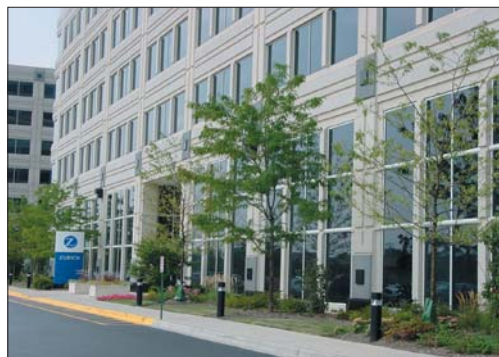
Bollards along drive.
