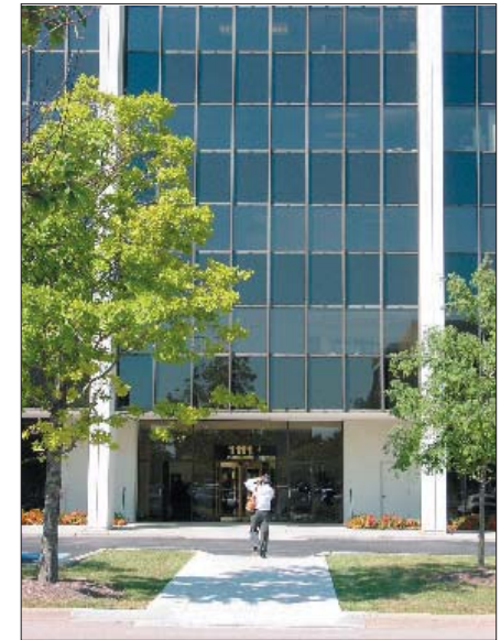
Pedestrian path in parking areas.
