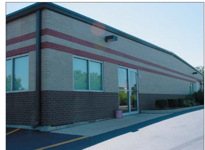
Entry is unattractive and difficult to find.
