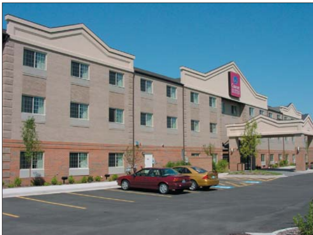
False facades are discouraged.
