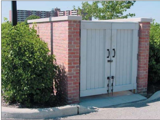
Refuse enclosure augmented with plantings.
