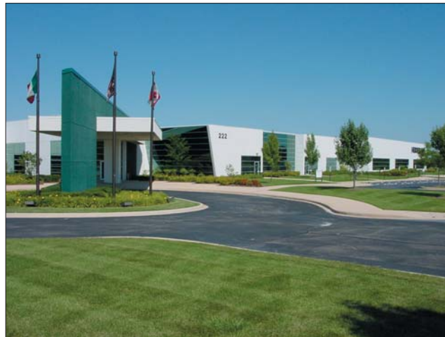
Office section of office/warehouse often provides opportunity for unique roof element and treatment.
