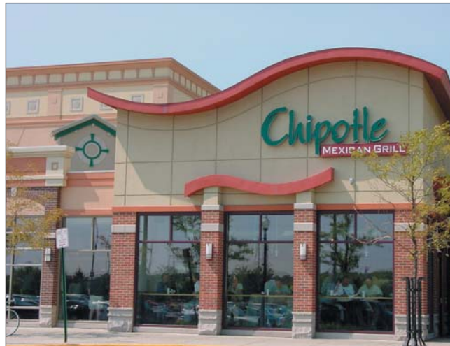
Building shape and color allude to the business name.
