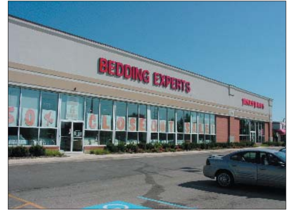
Site lacking clear pedestrian route from parking.
