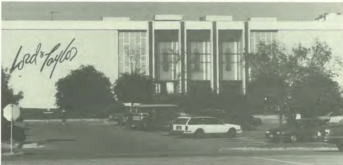
The Lord and Taylor store at Woodfield Mall, which was added to the original mall in 1973, will be refaced and structurally altered as a new retail wing as part of the proposed mall expansion. A new Lord and Taylor, Nordstroms and a two-level parking structure will be constructed on the end of the new wing. The expansion will add 450,000 square feet to the existing mall, bringing the total square footage to more than 2,700,000 square feet.
