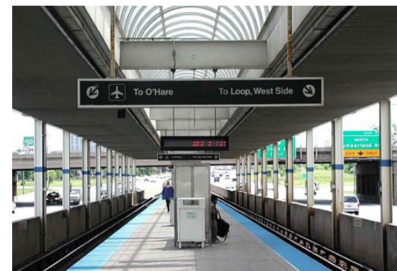
CTA station at Cumberland (Source- Chicago Transit Authority)
